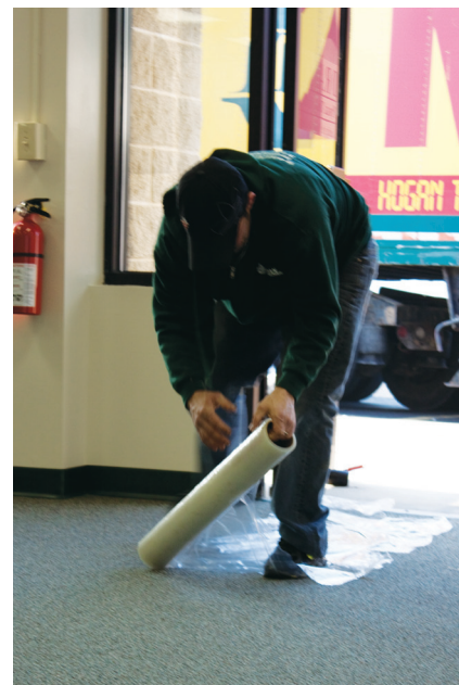
Clinic drywall and carpet protection.
